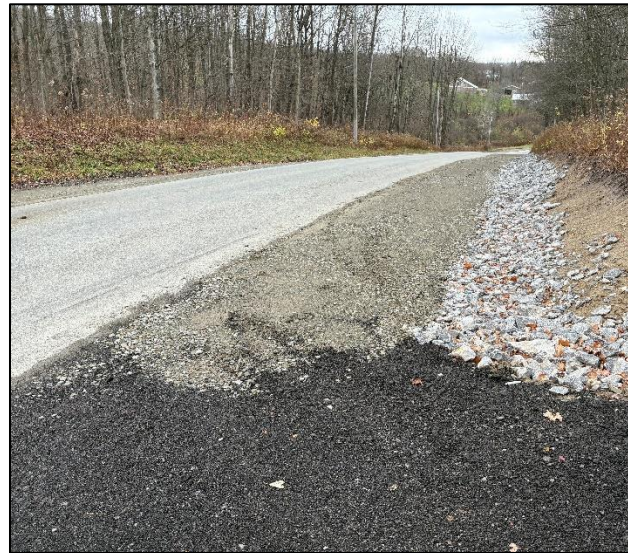
Photo of swale construction can be seen at Burdick Road.
