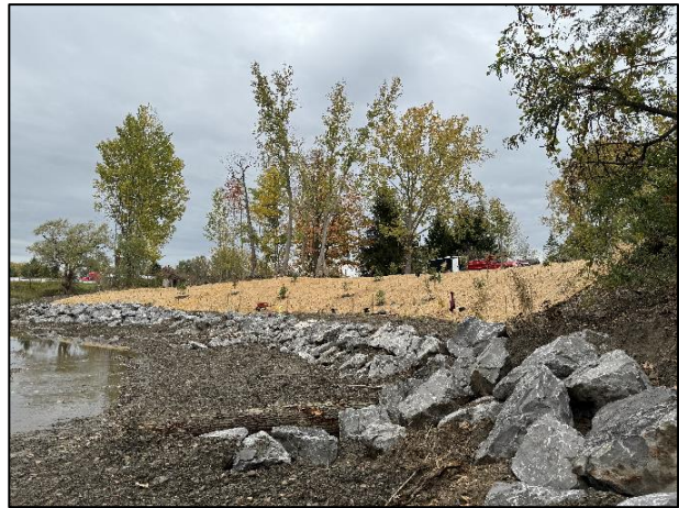
Photo 2. Ball Creek 10/11/23 after construction.
