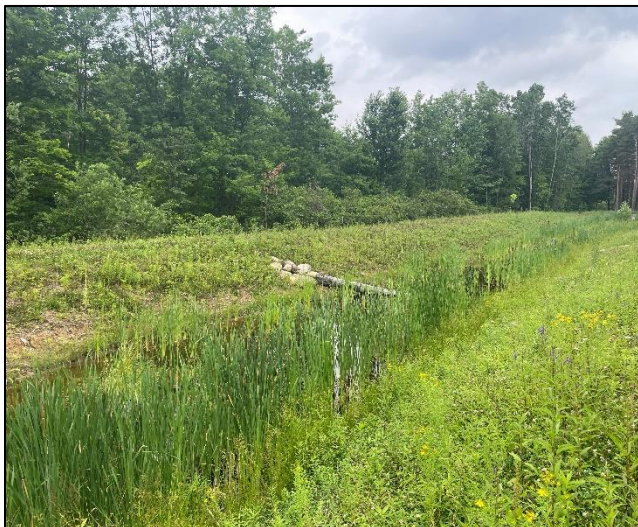
Photo of the western wetland pond after construction. A turtle basking log can be seen center frame.
