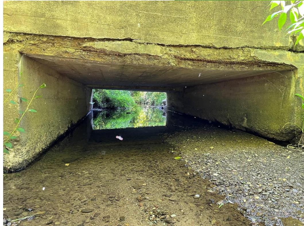
Pictured above is an aged culvert located on Elmwood Road. The structure has degraded significantly at the top and right of the frame. Stream erosion is also a concern.
