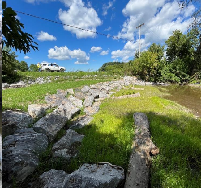
Pictured above is the Stow Road Bend after substantial completion, including a bendway weir pictured at the bottom right of frame.
