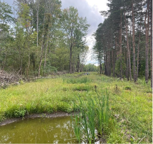
Photo of a new stormwater channel after construction.
