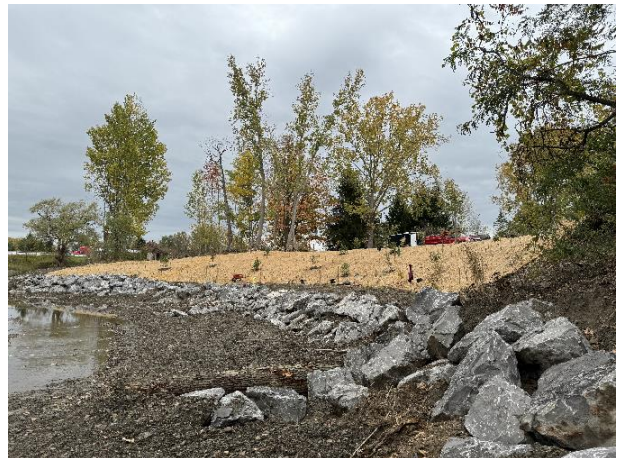
Photo 2. Ball Creek 10/11/23 after construction.
