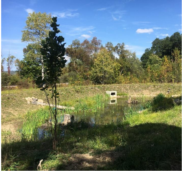
Photo of the east wetland pond after construction.
