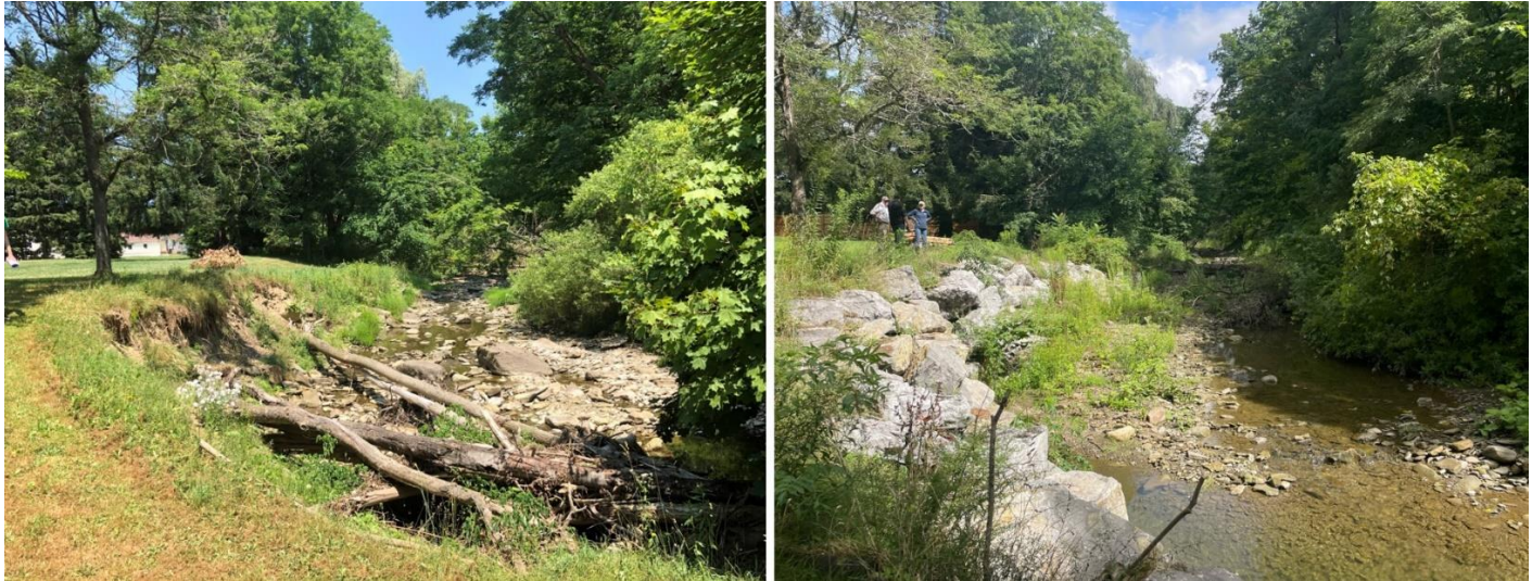
Figure 1. Pictured above is a stream stabilization project that was completed on Dutch Hollow Creek, at left is the bank in 2020 before construction. At right are members of the project team visiting the site in 2024.
