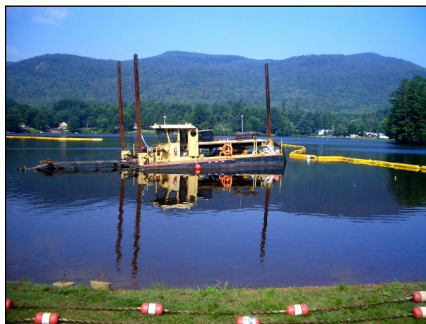
Figure 6-2: Lake Algonquin hydraulic dredging (Wells, NY)
