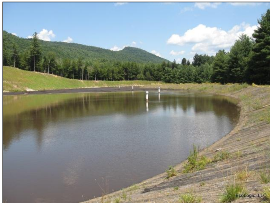
Figure 6-3: Sediment basin used for dewatering dredged material (Wells, NY)
